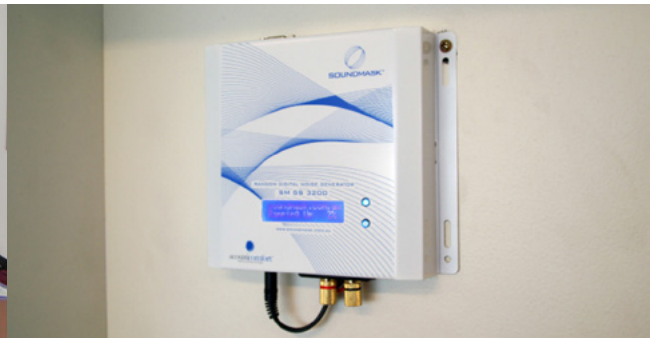
Soundmask's shelf generator SM-GS-3200 affixed to wall
